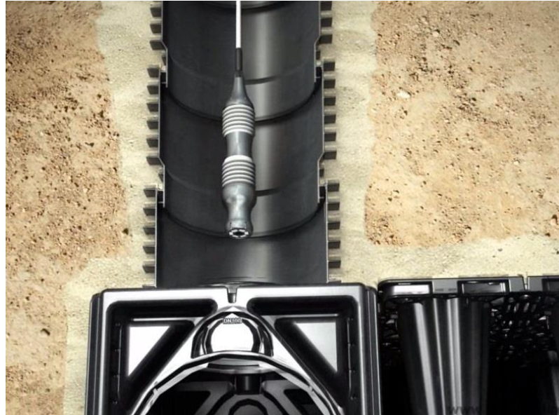
Camera access down access shaft
