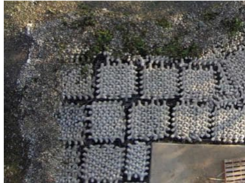
PIER SCOUR PROTECTION
