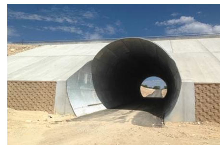
STEP-BEVELED END WITH CONCRETE
