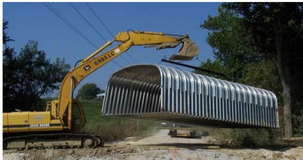
LIFT AND SET IN PLACE
