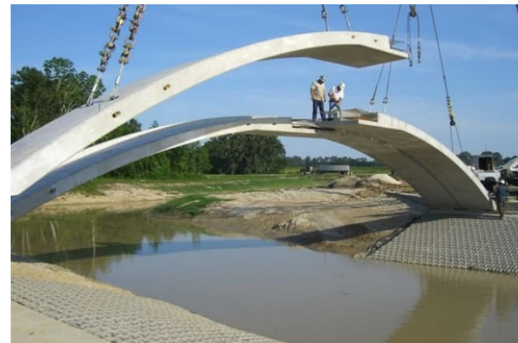
TWIN LEAF CONSTRUCTION
