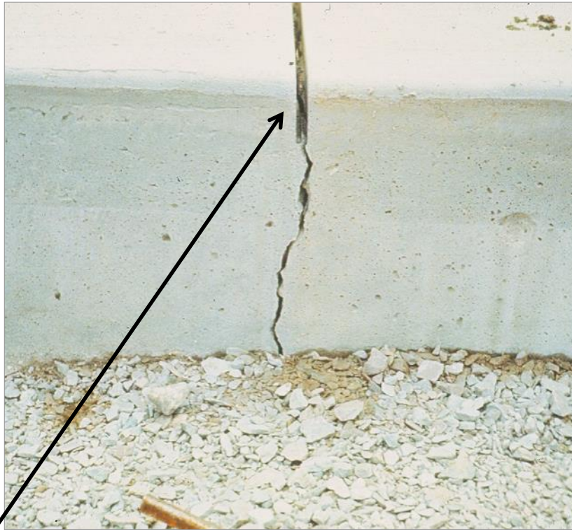
This joint was sawed at correct time
