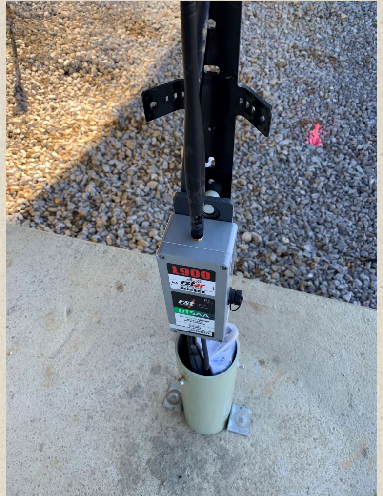
Completed Shaft Install
