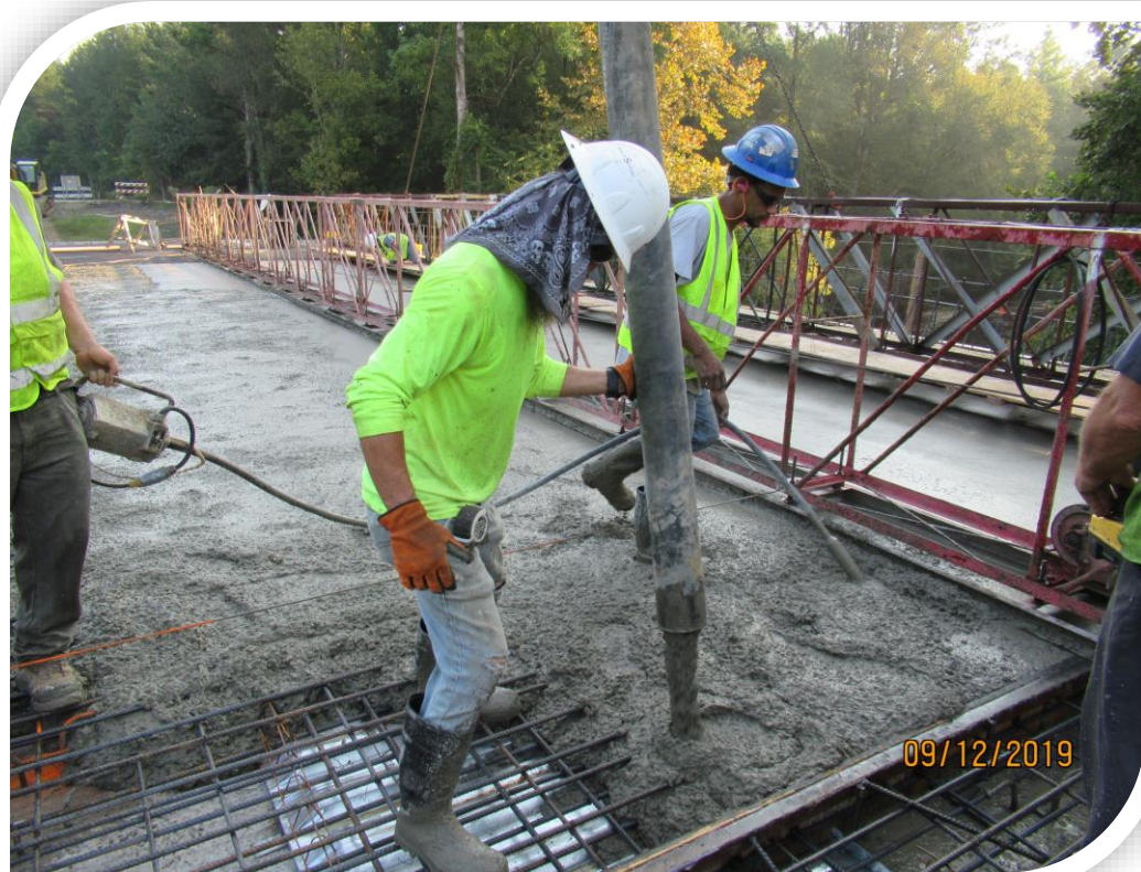
Placement of Concrete Superstructure
