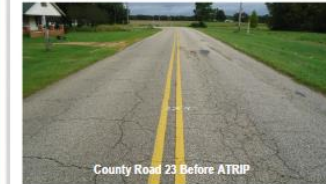
County Road 23 Before ATRIP
