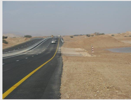
Irish passage after installation – fully functional, no erosion
