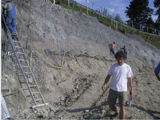
Stage 1: Anchoring the 3D grid
