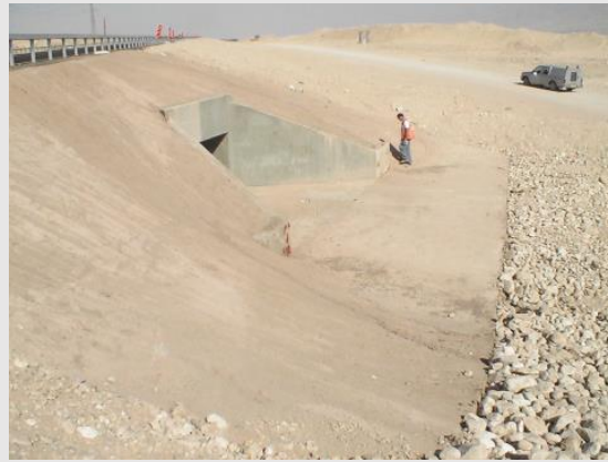
Protecting soil erosion in culvert areas – before & after
