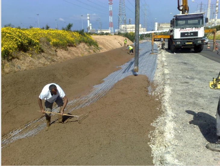
Rigid lining of ditches & canals
