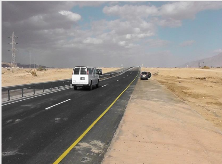
Culverts & "dip" areas
