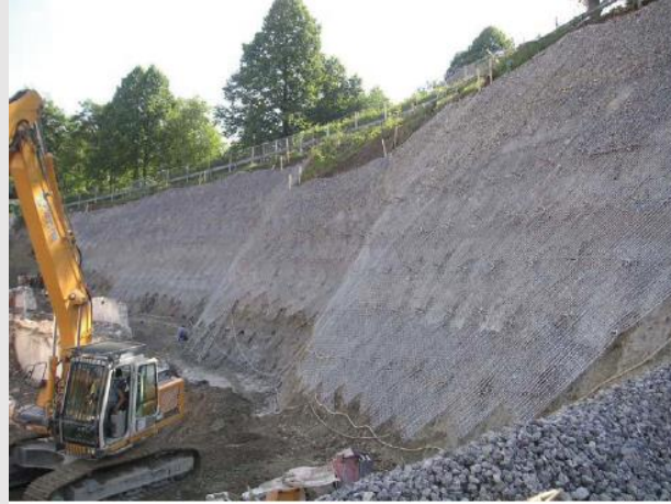
Stage 2: spreading stones & soil mixture
