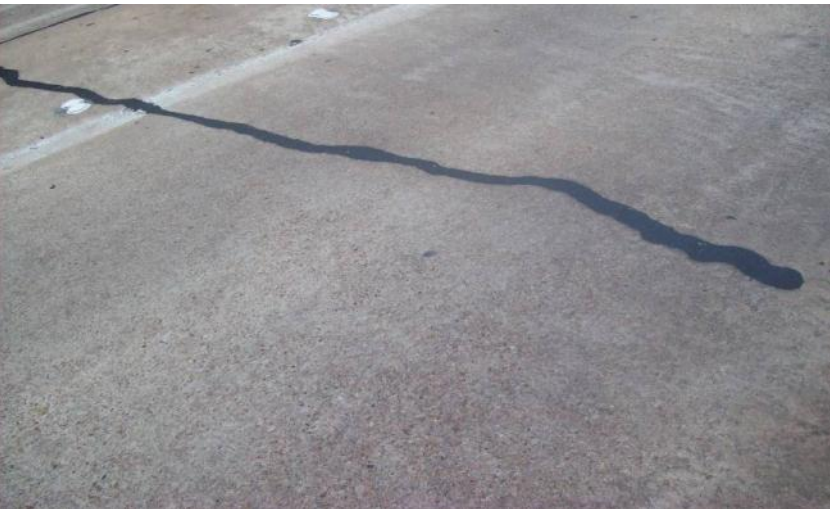
Crack Seal
