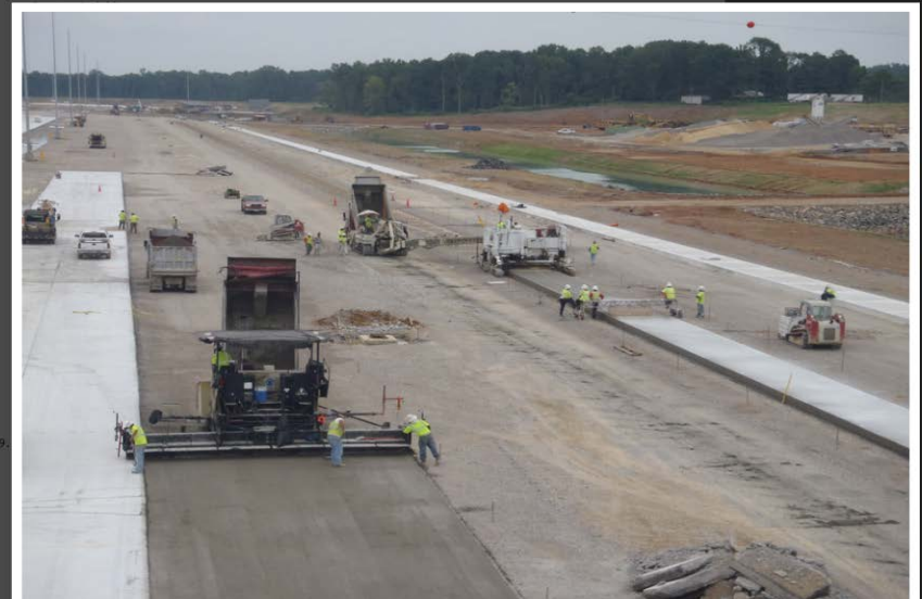
RCC and PCC Installation Image 1 of 3
