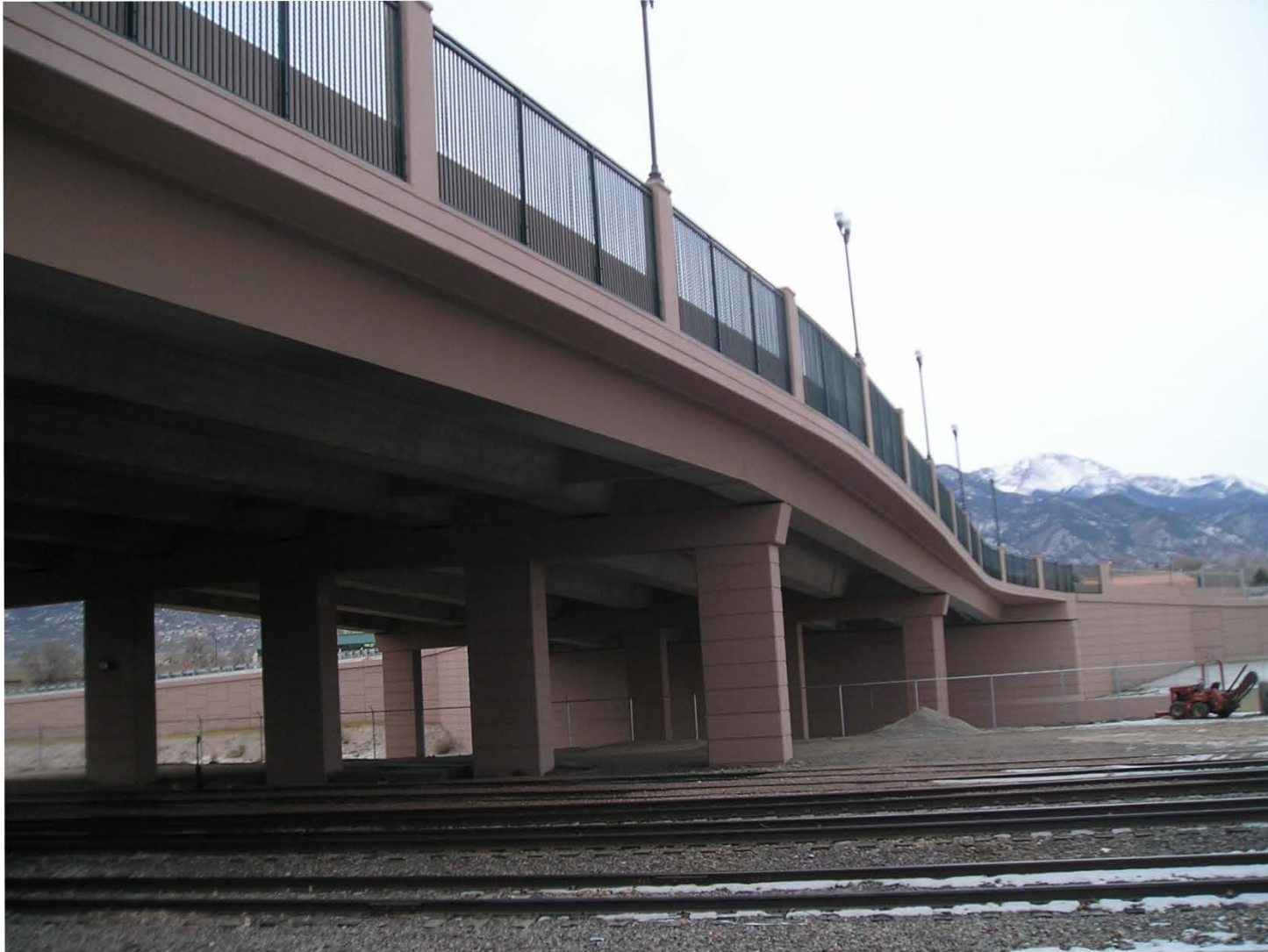
Bijou Street Bridge
