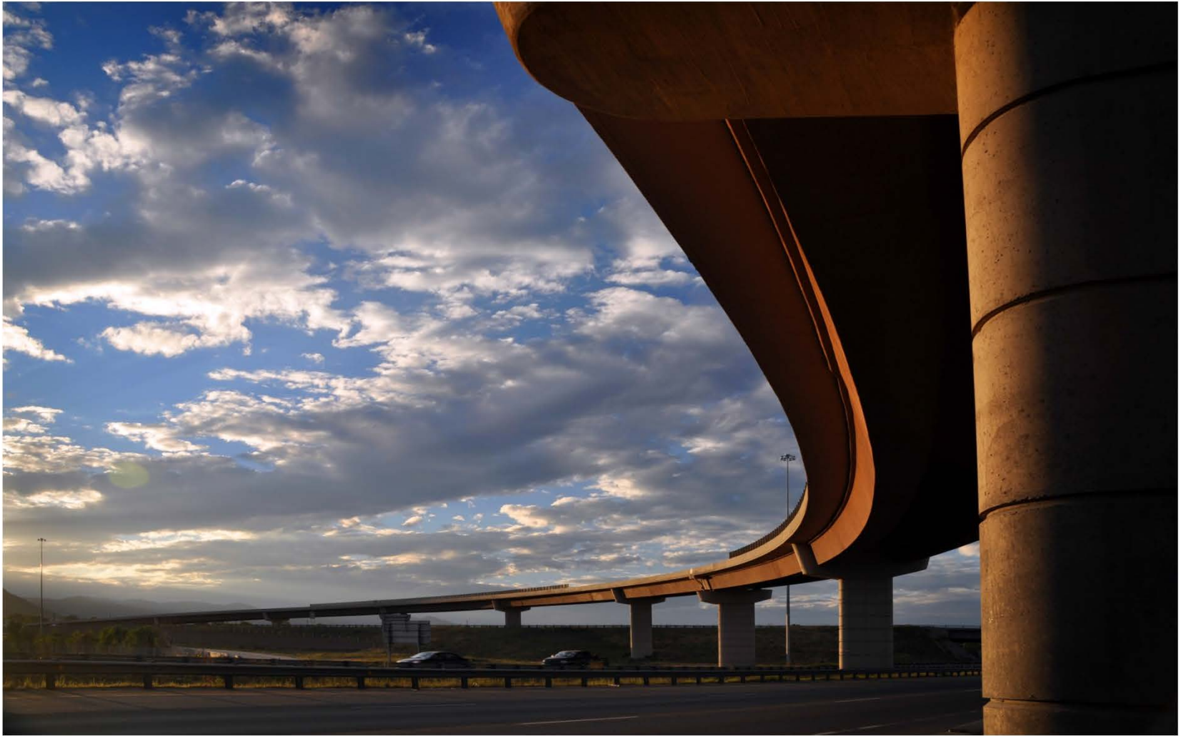
SH 58 Ramp A
