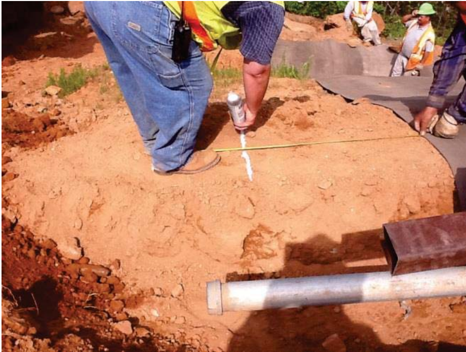
Spray marking for the right side anchor trench
